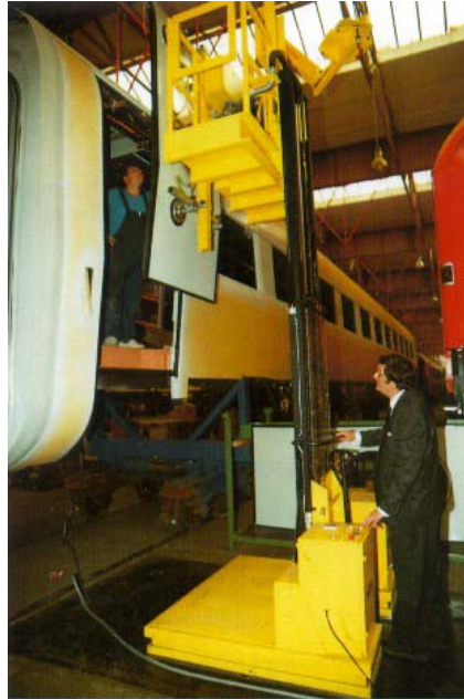
Fig. 3: Door and window assembly aid using the omnimobility of an air-cushion gear
